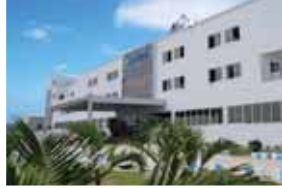
Rudrapur Plant (Green Building)
